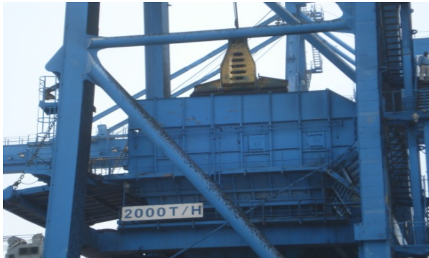
Coal unloaded from the ship and put into hopper
