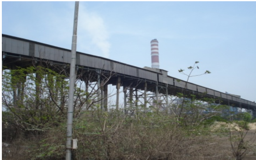
Closed elevated conveyor system
